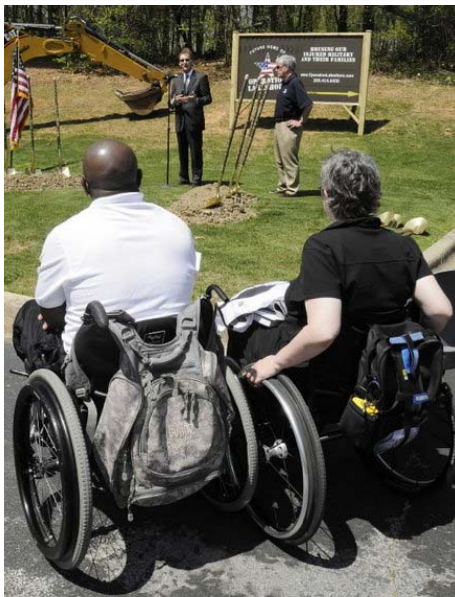
W.D. Foster of Alabaster, left, and Dr. Leah Hagedorn of Norfolk, Va., watch today's groundbreaking at Lakeshore. (Beverly Taylor/Birmingham News)
